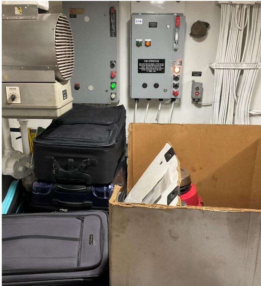
Excess equipment and storage. Note the space heater to the left within inches of cloth luggage. Everything is blocking electrical breakers. If there was an electrical fire it will not be easy to reach the breaker safely to secure power to that system. (Photo Credit: Mr. Robert Penner)
