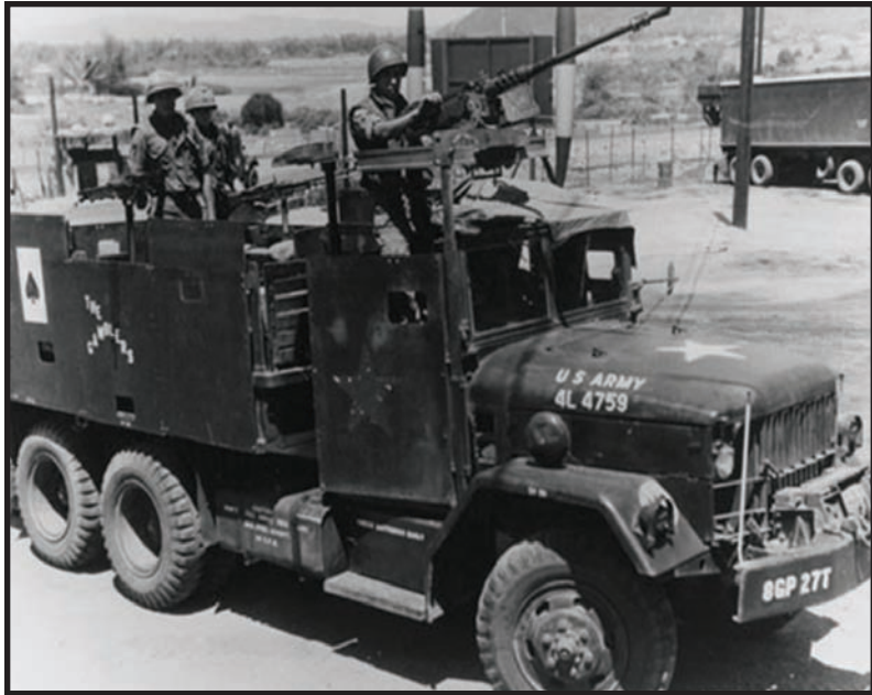
Figure 6. 8th Group 2 1/2-Ton Gun Truck with Steel Plates. This truck has sandbagged floors and two pedestal-mounted M-60 machine guns.
